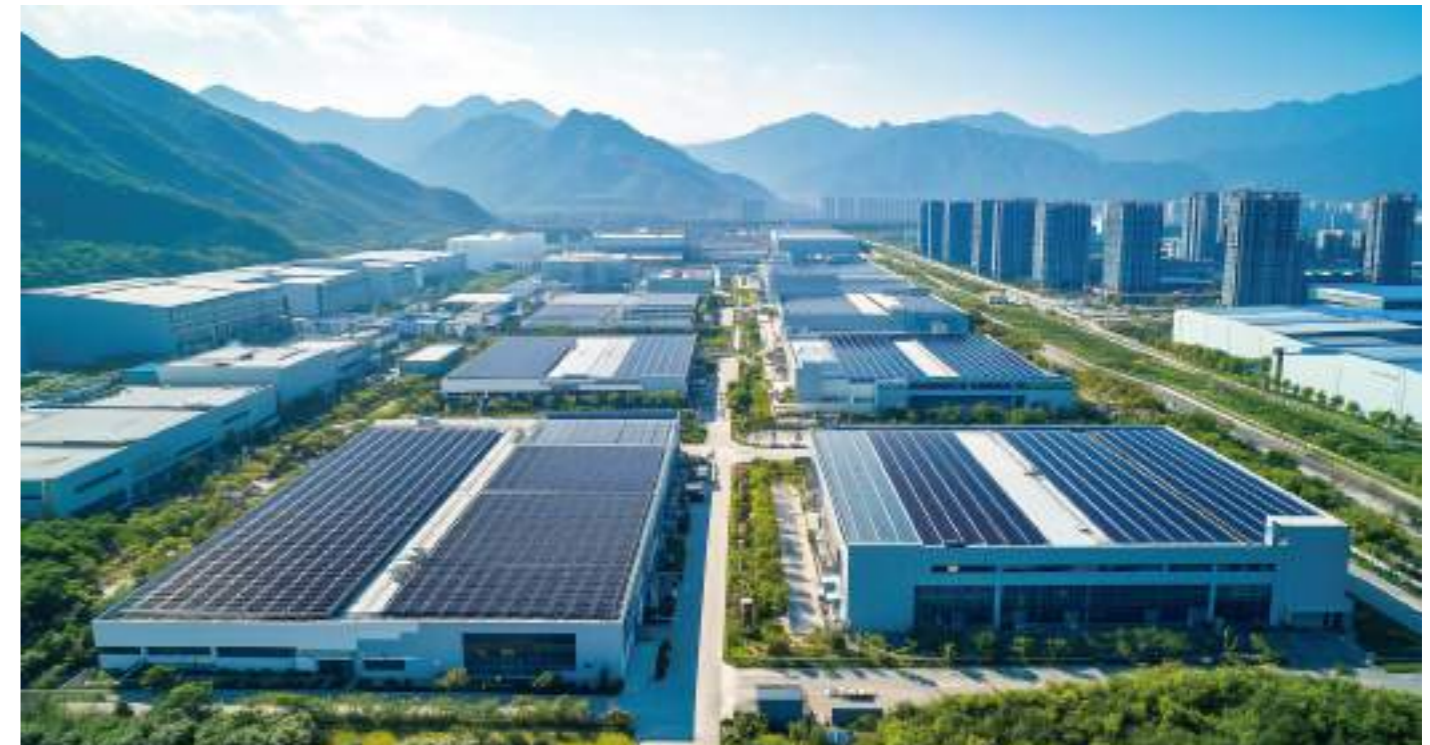
Mountain Energy Storage Deployment (2MWh)
